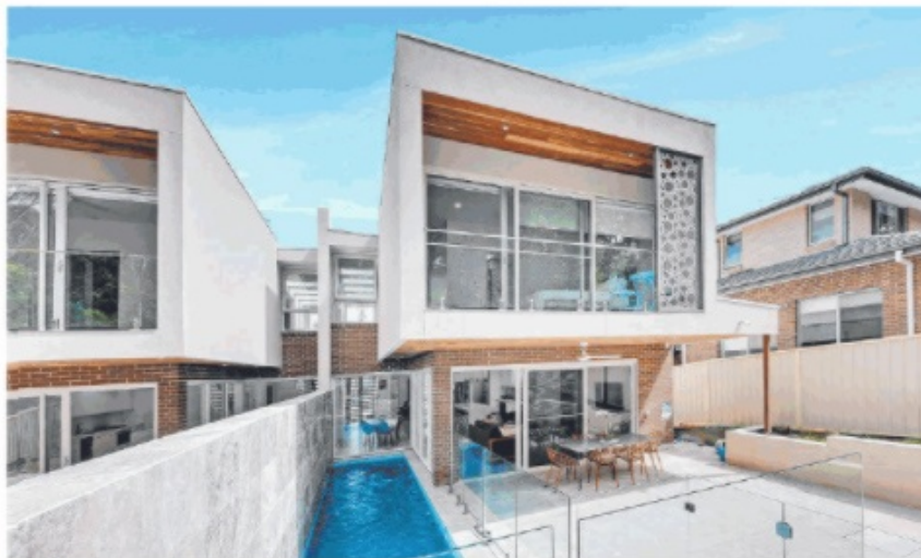
The thick stone wall alongside each of the lap pools separates the twin duplex properties
